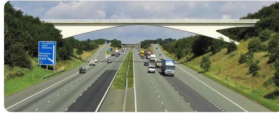
M1 motorway in Yorkshire
